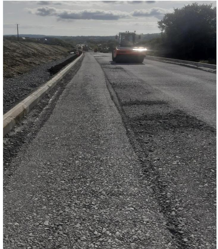
Looking towards Black Lion Road from Norton Road, the picture features approximately 500metres of type 1/sub-base in preparation for tarmac. As seen in the picture on the right, the kerbs along the carriageway have been completed. There are many different types of road kerbs used and those featured are standard barrier HB2 and mountable splay kerbs designed for different purposes.
