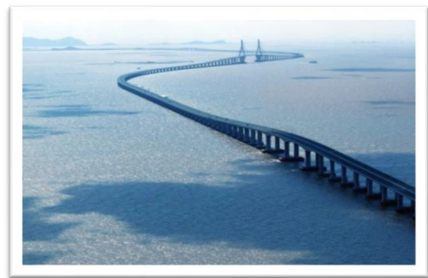
HANGZHOU BAY BRIDGE
