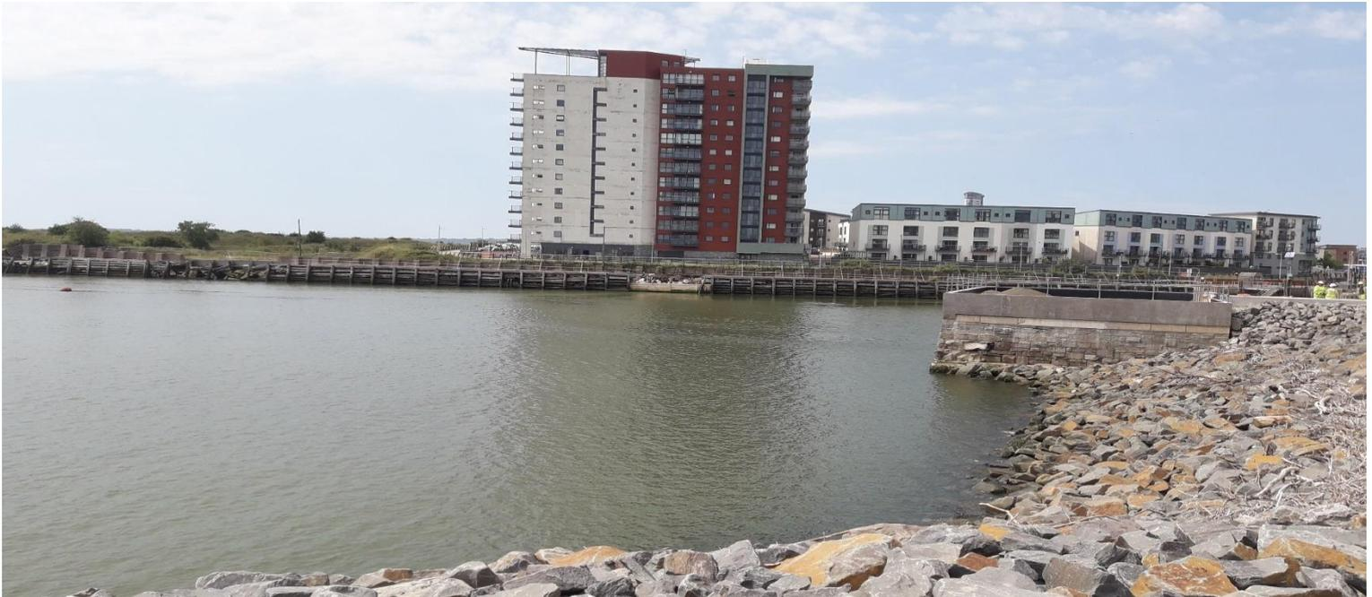
Works to the promontory featured in the right-hand side of the above photograph has been reinforced with over 12 tonnes of steel and the walls are formed using 67m<sup>3</sup> of concrete. Where possible Griffiths employees work at SA1 with local contractors and suppliers appointed to support on site activities. As at other areas of SA1 benches and street furniture will complete the aspect of this area which in the future can be used as a viewing platform.
