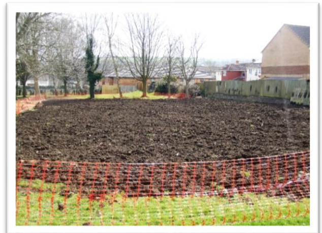
Photo taken 6th April 2016 after groundwork
