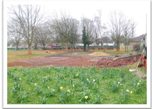
Photo taken 29th March as work begins
